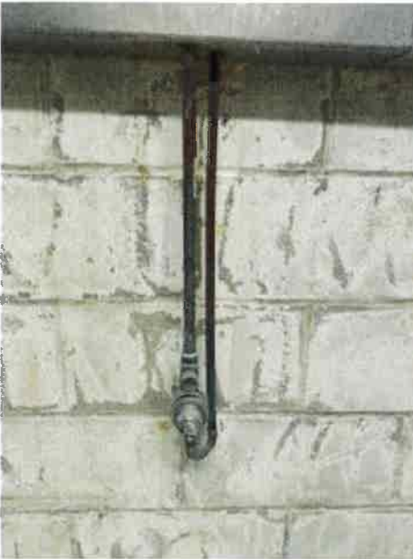
Replace shower manifolds
