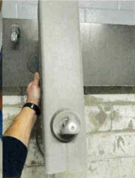
Replace shower valves
