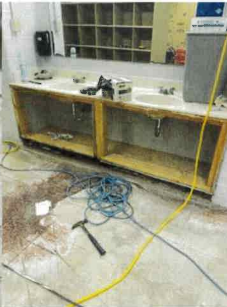
Replace men's & women's locker room sinks
