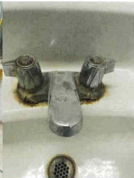
Replace sink fixtures
